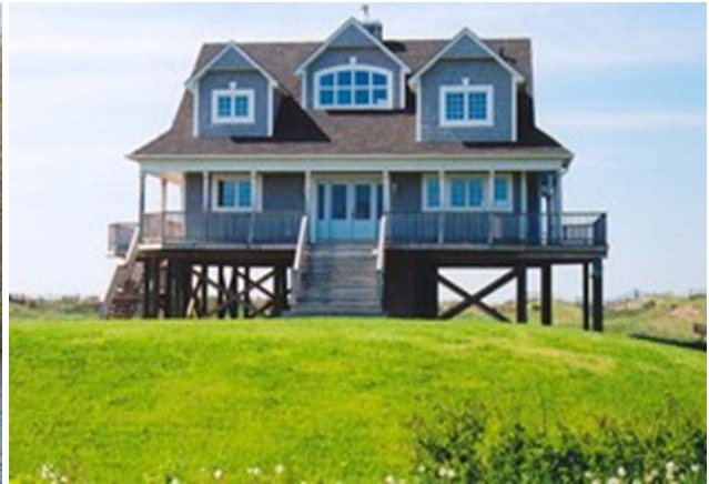
An oceanfront home on piers in Robichaud, New Brunswick
